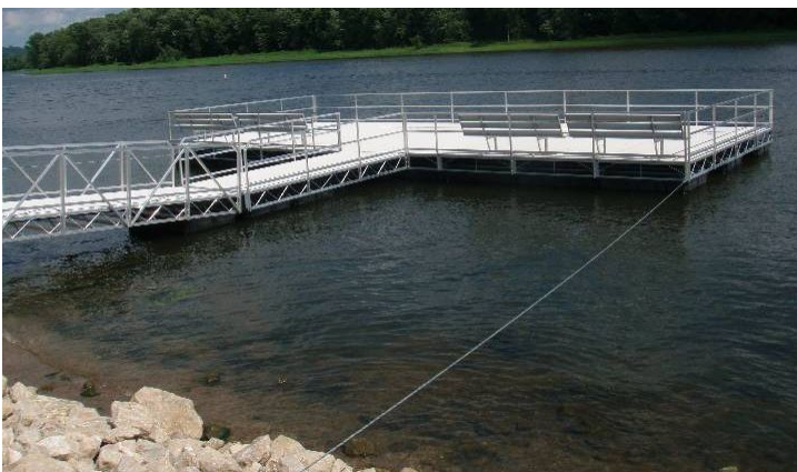
The platform will include an open section housing the aerator and will be lit from above with a lighting source.
